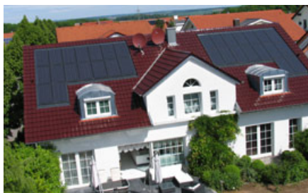
Photovoltaic in-roof system SOLON Black; Modules with black frame and black side panels. Photos: SOLON SE
