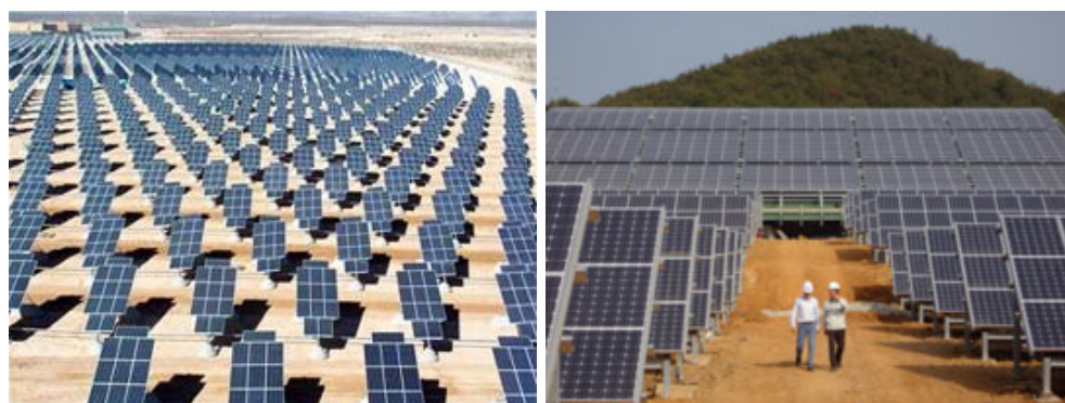
Left: North America's largest solar photovoltaic power system with 70,000 solar panels on 140 acres of unused land at Nellis Air Force Base (Nevada). Right: Solar power plant by SunTechnics in South Korea with an output of one megawatt. At SinAn, southwest of the Korean capital Seoul, a new sun-tracking photovoltaic system with a total maximum output of 19.6 megawatts is under construction. Pictures: US Air Force; SunTechnics.
