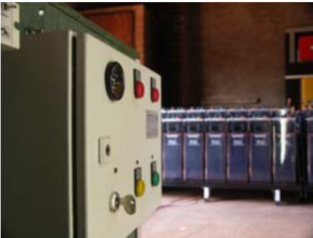
Generator control panel (left foreground). About two dozen batteries guarantee power supply around the clock. Photos: Energiebau Solarstromsysteme GmbH
