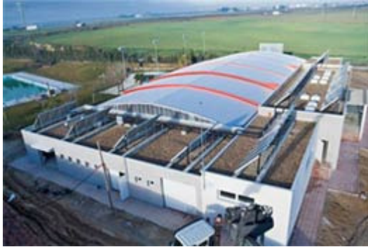
Solar thermal systems on a sports hall in Ugena (Toledo) and a hotel in Almería. Photos: ASIT Solar (AURA SOLAR; SNELL SERVICIOS GLOBALES)
