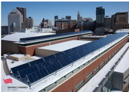
Megawatt-Solarthermie-Anlage in St. Paul, Minnesota
